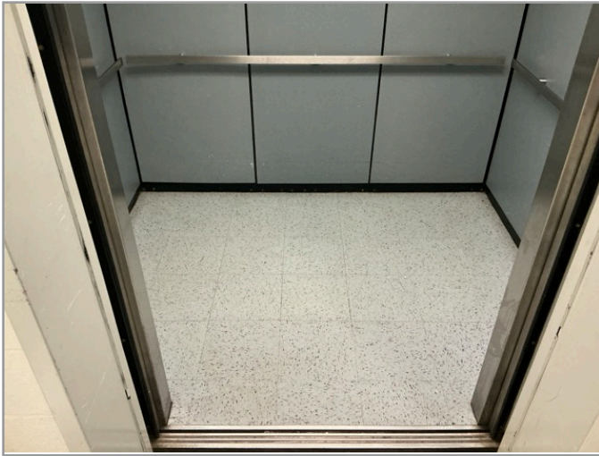
LOBBY LOOKING AT CABS (WITH DOORS OPEN)
